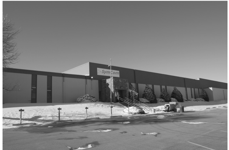
SymCom's new building located on Disk Drive in Rapid City, SD.
